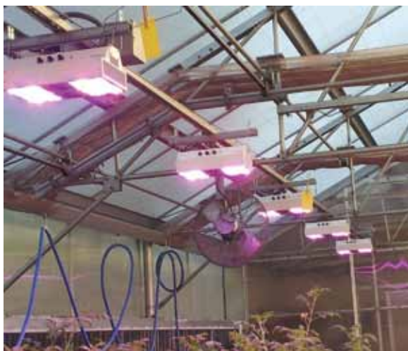
Replacing aging HID lights with LED lights is an effective strategy for increasing light while decreasing energy consumption and costs. Author Kevin Wells is depicted in the above photo of a greenhouse in the Northwestern United States.
